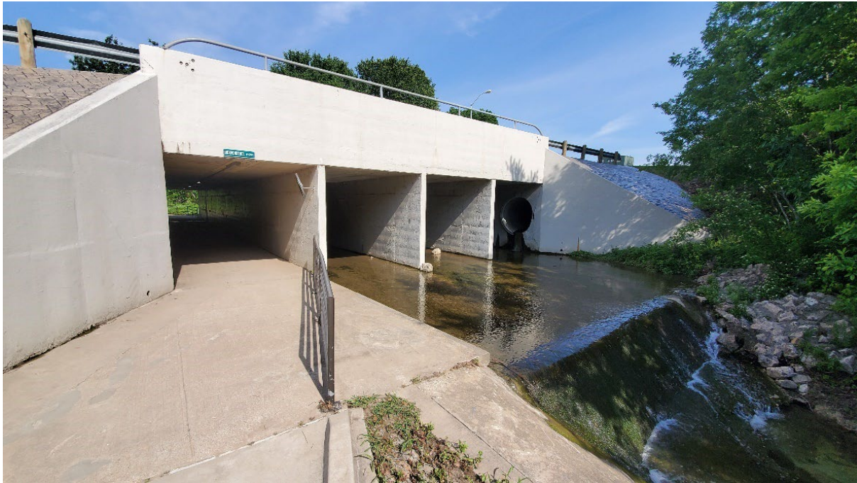
Figure 2.52: Staged or Tiered Culvert Design Used in North Texas with Multiple Culvert Sizes and Flow Elevations
