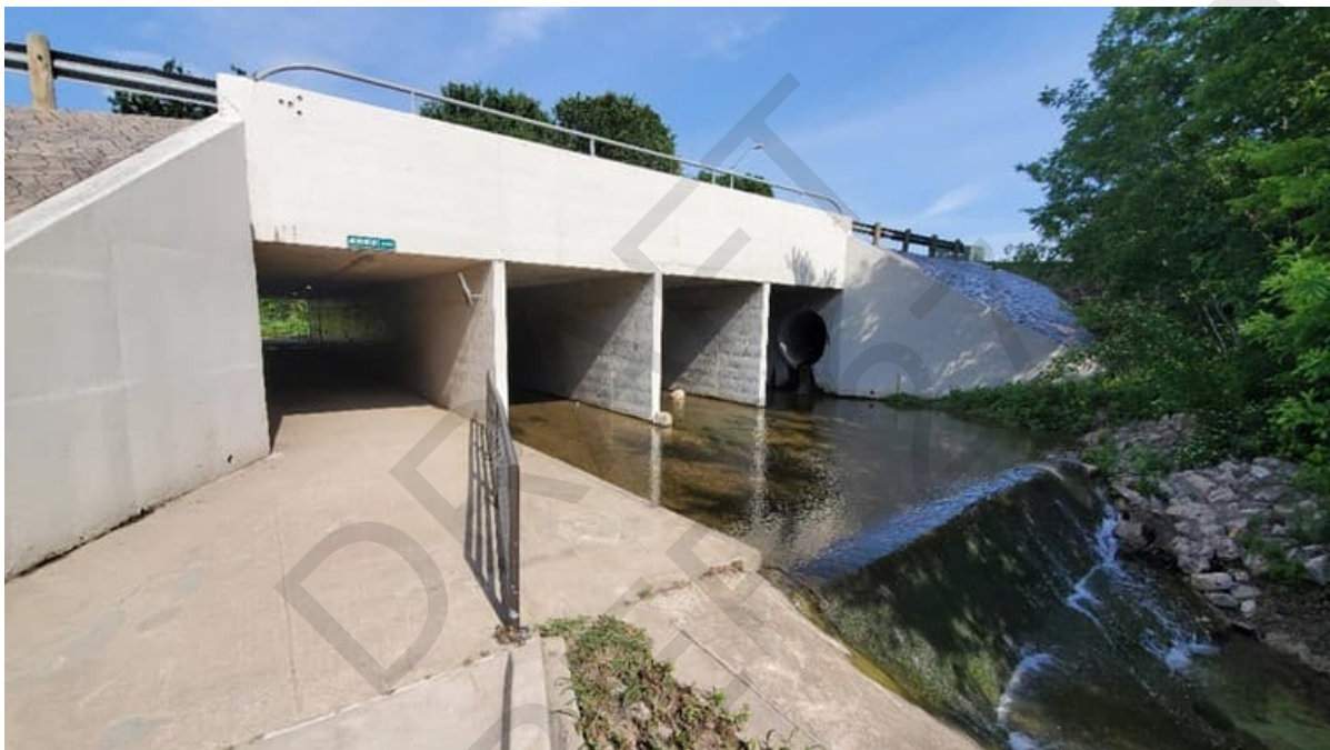
Figure 2.48 Staged or Tiered Culvert Design Used in North Texas with Multiple Culvert Sizes and Flow Elevations
